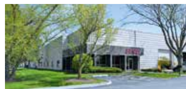
Sales office in Chicago becomes a full production facility
